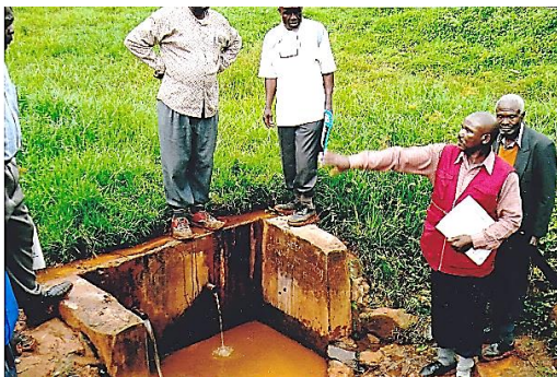
The Water Committee visits a renovated spring
